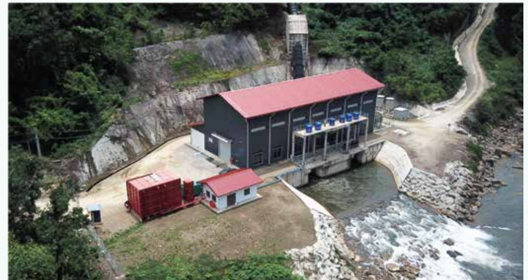
Visual 4: Telekosang Hydro One power plant
